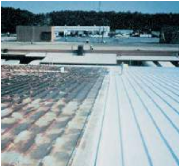
After Year 21, roof restoration is another option if the roof has been well maintained.
